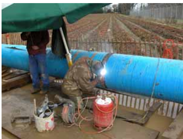
Two pipe lengths were welded together.
