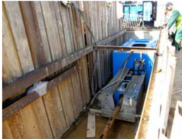
The GRUNDOBURST with 2,500 kN (250 t) pulling force is the largest pipe burster available from Tracto-Technik.
