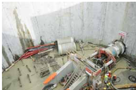
The jacking station built inside the 25 m diameter storage basin.
