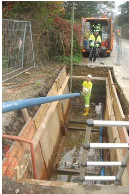
The ZMU drinking water pipes being brought in.
