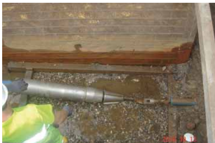
The cutting and expansion head and the bursting rods ready for a bursting run.
