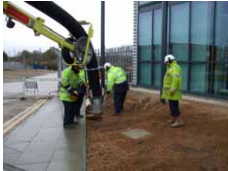
TT-UK/RSP Suction Excavator operator training taking place at National Grid’s training academy in Hitchin.
