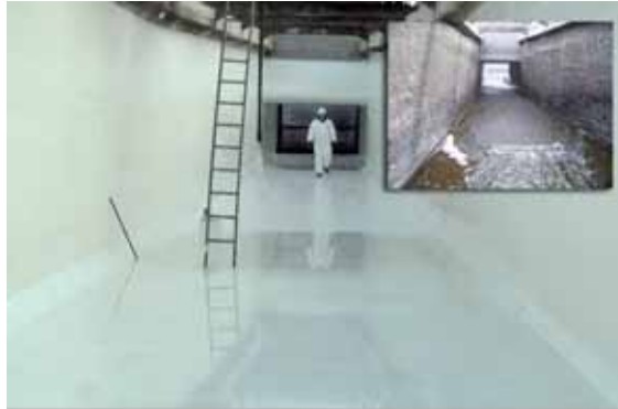
Before and after the application of Ultracoat at the Liawenee Flume.
