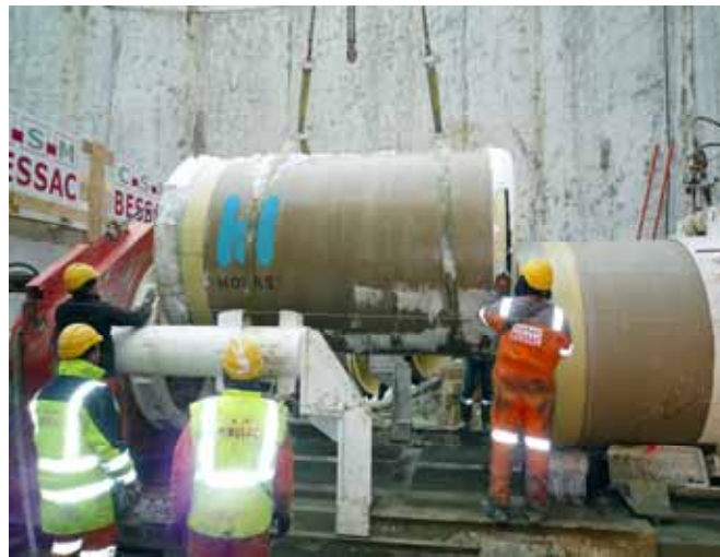
HOBAS flush jacking couplings provided a leak-tight line.
