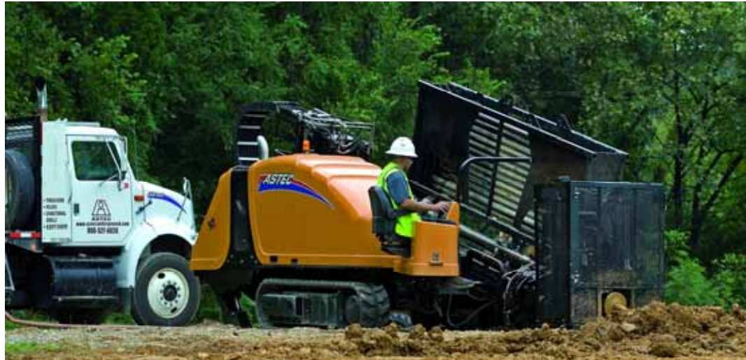
The new Astec Underground DD-4045 horizontal directional drilling rig.
