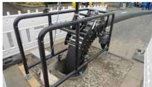
Long pipe installation using the Burstform technique through an existing manhole.
