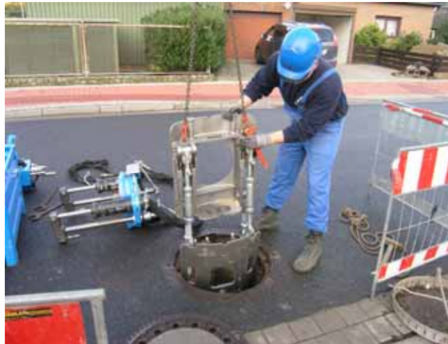
The components of the Grundobore 200 S make installation into the existing main pipe manhole simple.
