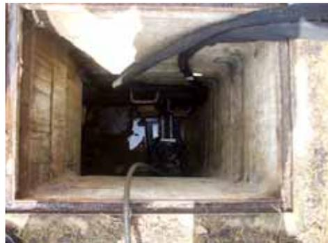
*The PB15 and its Docking Station in a 2.5 m deep manhole.*
