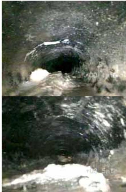
*Typical Pitch Fibre Pipe deformation at the Roakes Avenue site.*
