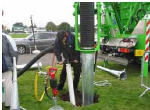
*An MTS Vacuum Excavation System from U Mole.*
