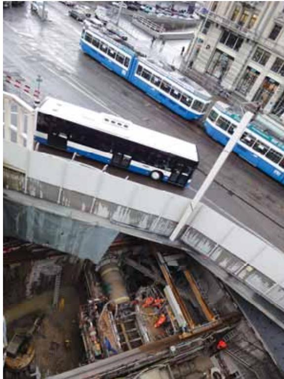
*HOBAS CC-GRP Jacking Pipes were installed as static pipe construction to prevent the buildings and streets above from subsiding.*
