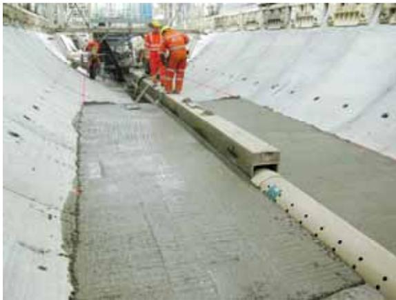
*DN 400 drainage pipes were installed in the centre of the tunnel floor and were cast in concrete to 180°.*
