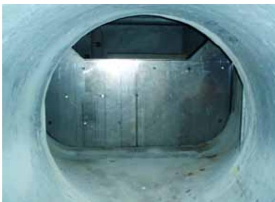
Made by Uhrig, the system uses modern flow monitoring techniques and automated control systems triggered by the flow monitoring systems to open and close the sluice gates as flow volumes in the pipeline change. This allows the pipe upstream of the sluice gate to be used as an immediate 'short-term' flow storage facility, with flows
